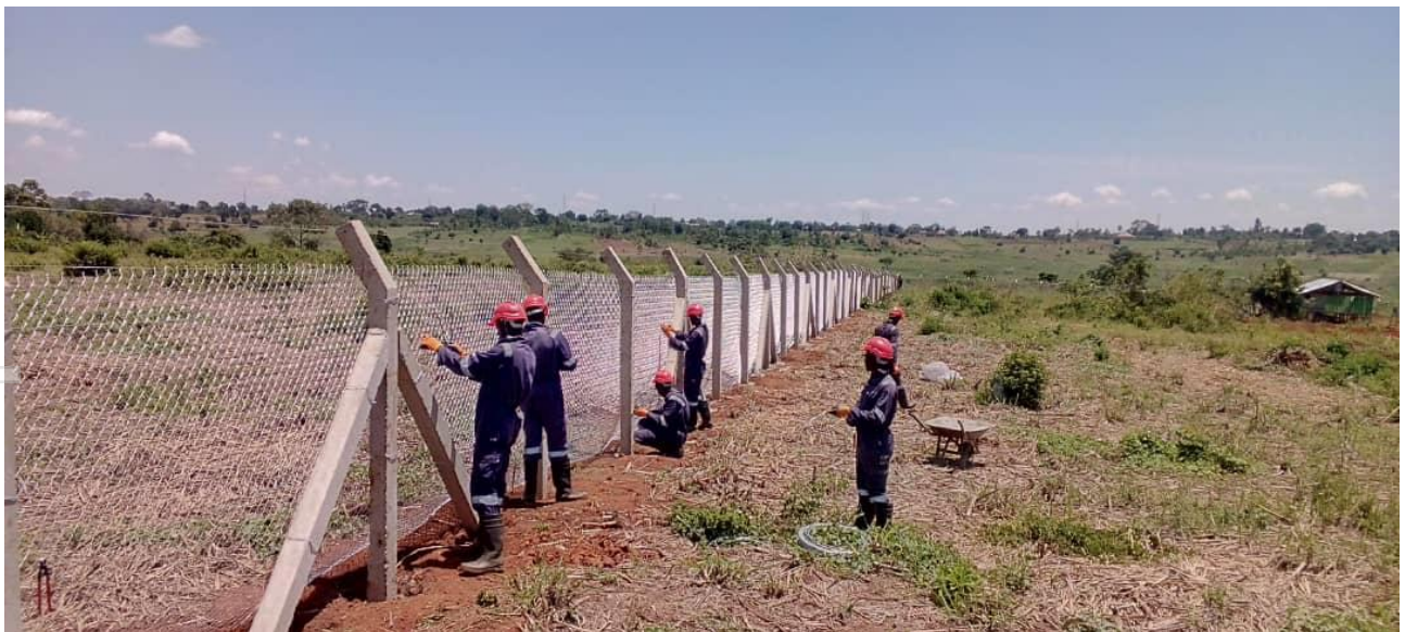
Figure 13: Boundary fence installation.
