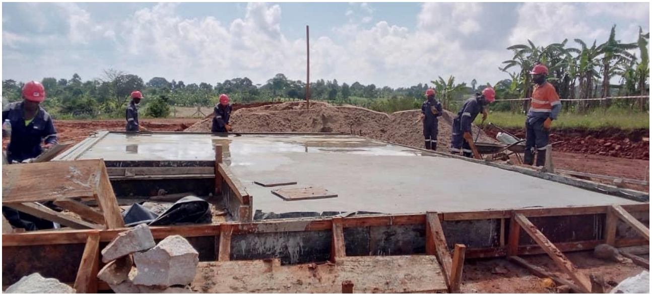
Figure 10: Agglomerator pad concrete slab poured and curing.
