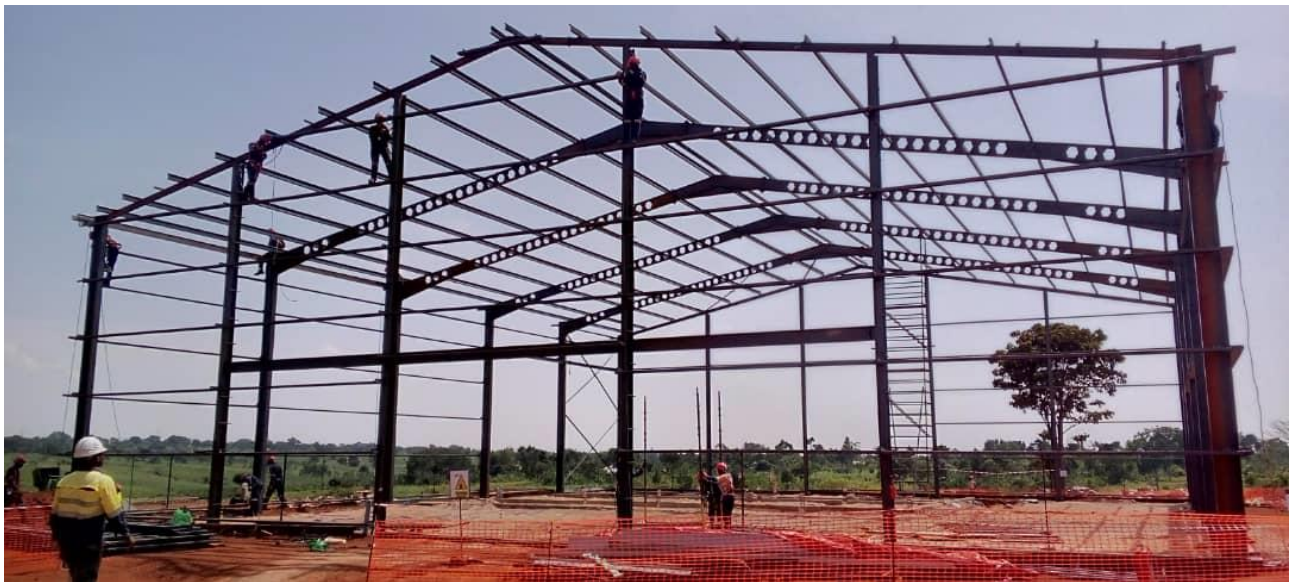
Figure 9: Makuutu Technical Facility frame structure erected.
