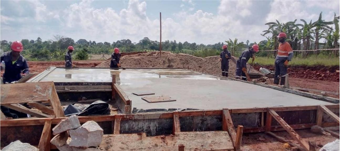
Figure 10: Agglomerator pad concrete slab poured and curing.
