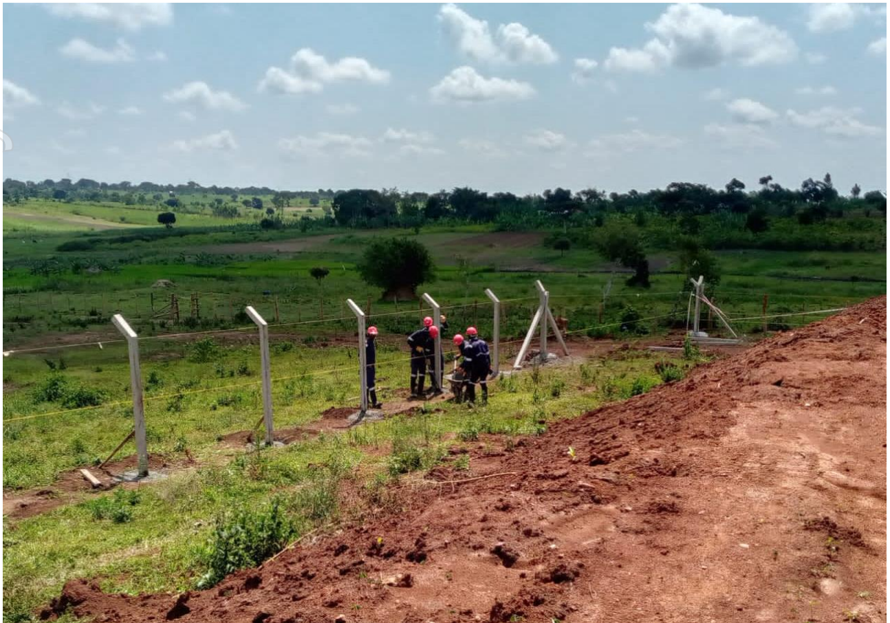
Figure 12: Installing boundary fence posts.
