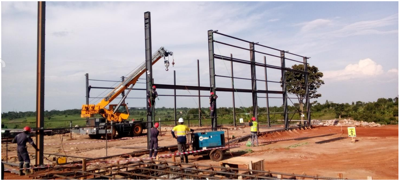
Figure 8: Erection of the Technical Facility steel column structure.
