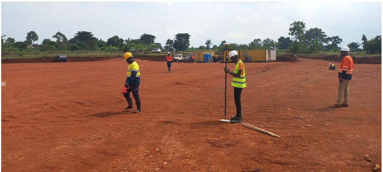
Figure 5: Marking out the Demonstration Plant footworks.
