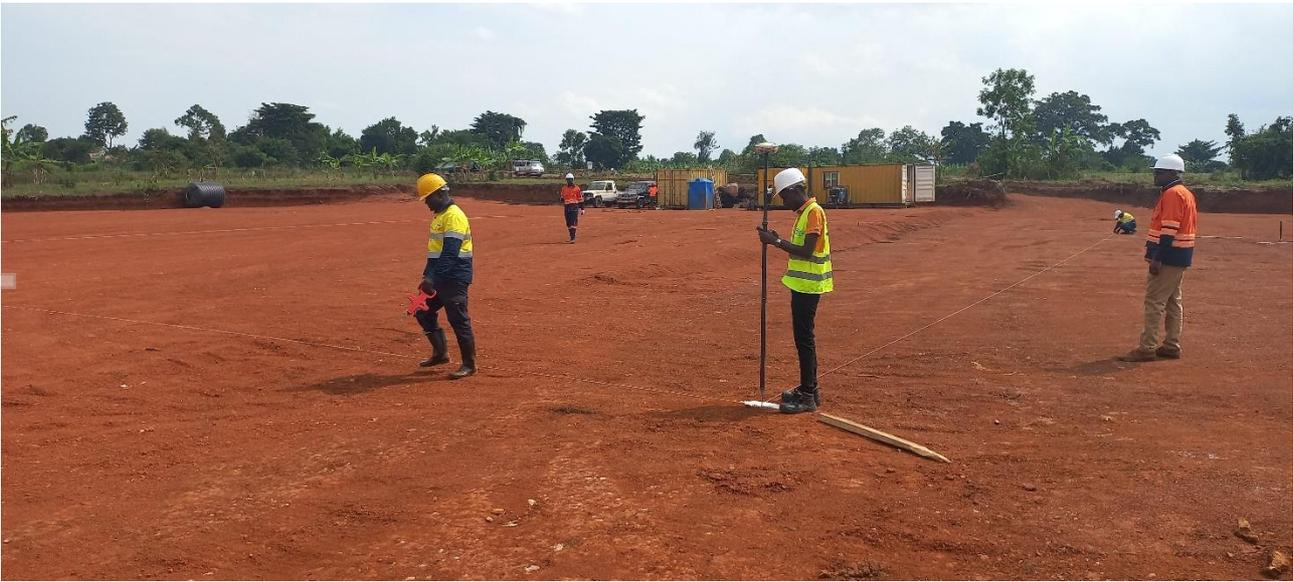
Figure 5: Marking out the Demonstration Plant footworks.
