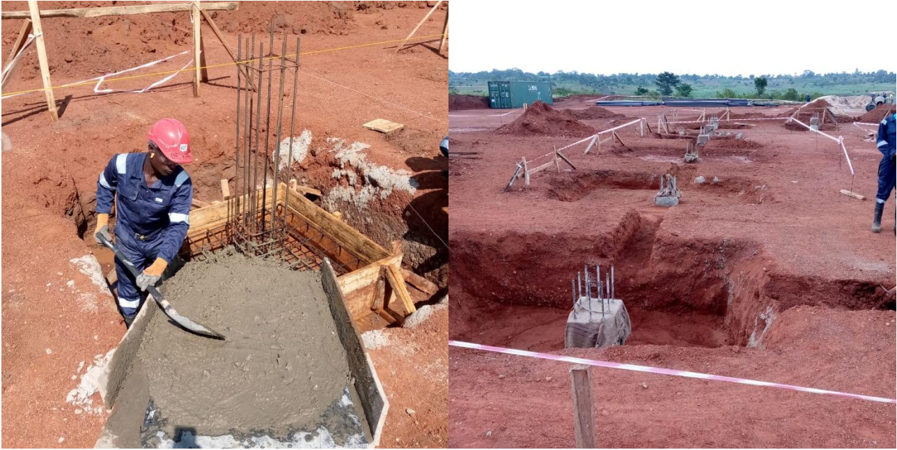
Figure 6: Casting of ground bases, on left, and excavations for the ground beam on right.
