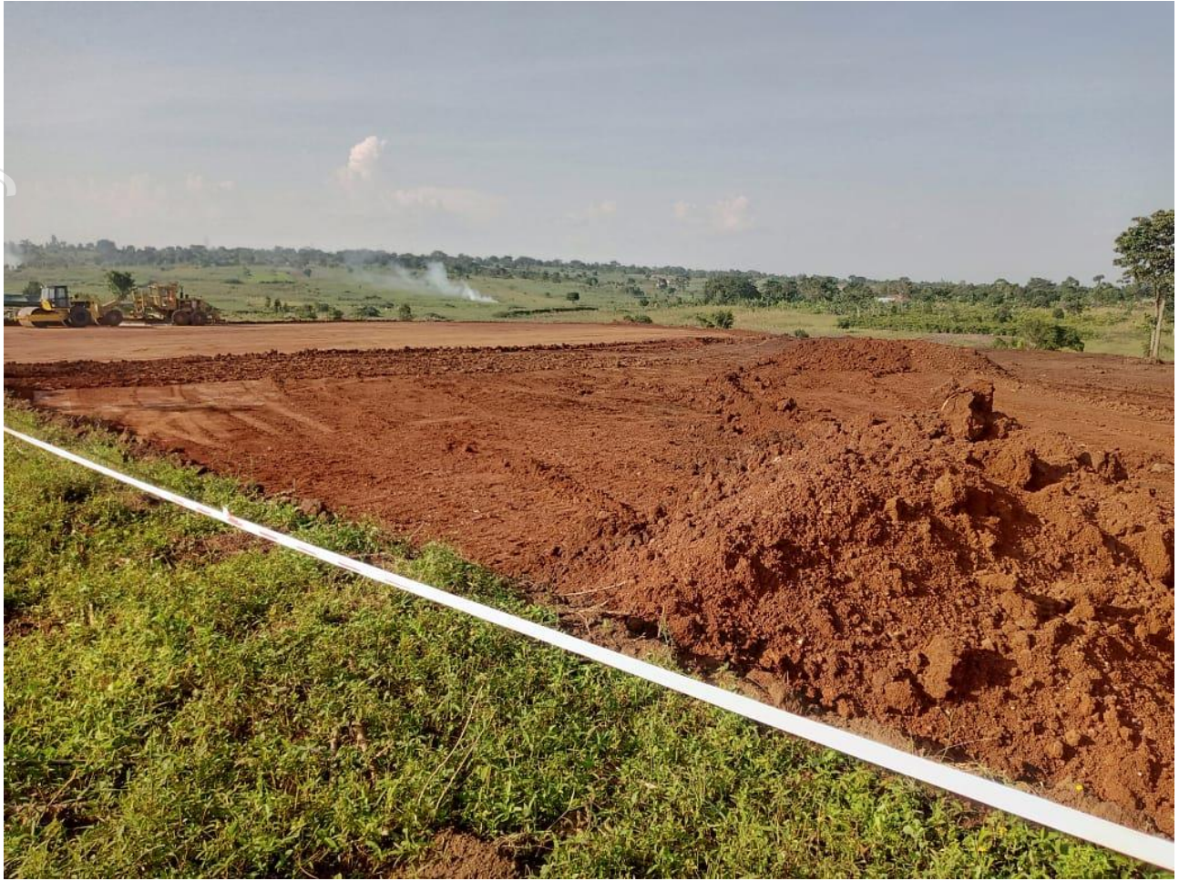
Figure 4: Removal of the topsoil layer across the Demonstration Plant facility area.
