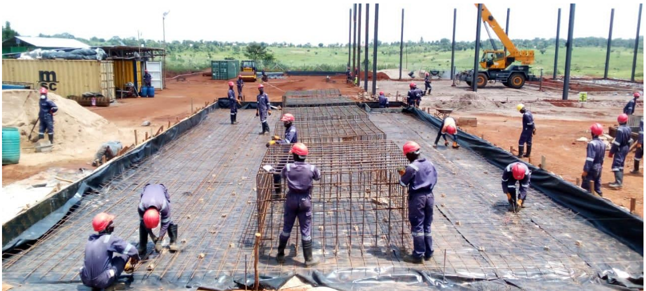
Figure 11: Heap desorption crib foundations prior to concrete pour.
