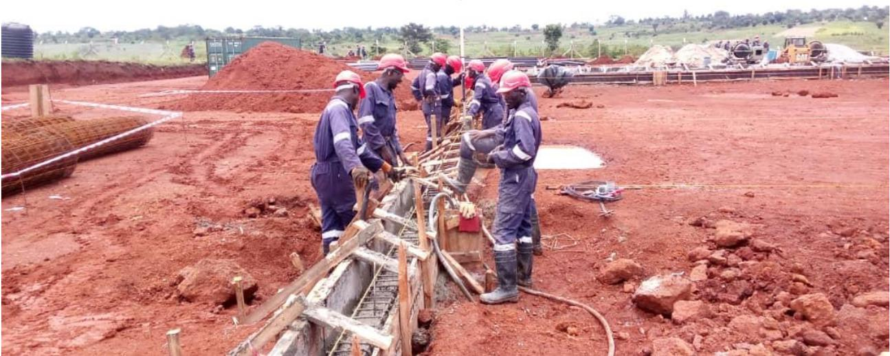
Figure 7: Casting of the Technical Facility ground beam.
