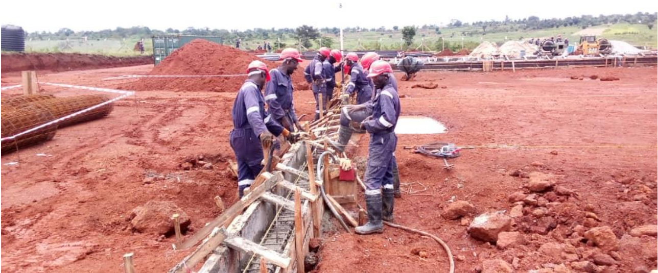
Figure 7: Casting of the Technical Facility ground beam.
