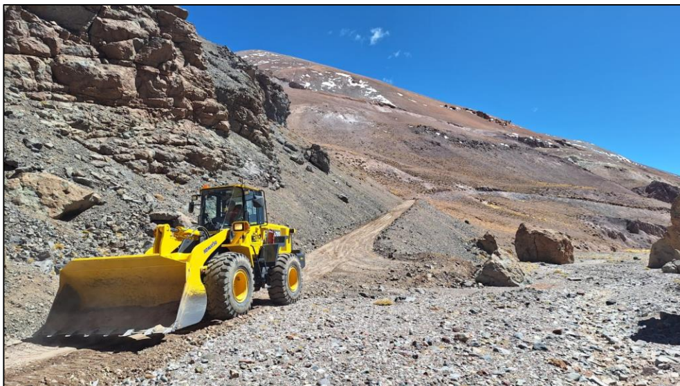
Figure 6: Earthworks machinery at the TMT Project
