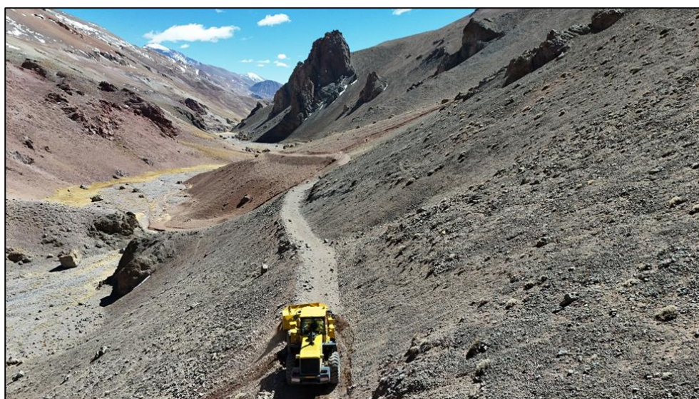
Figure 7: Drone shot capturing the restoration of the access track, track condition is prior to the first pass light vehicle upgrade works.
