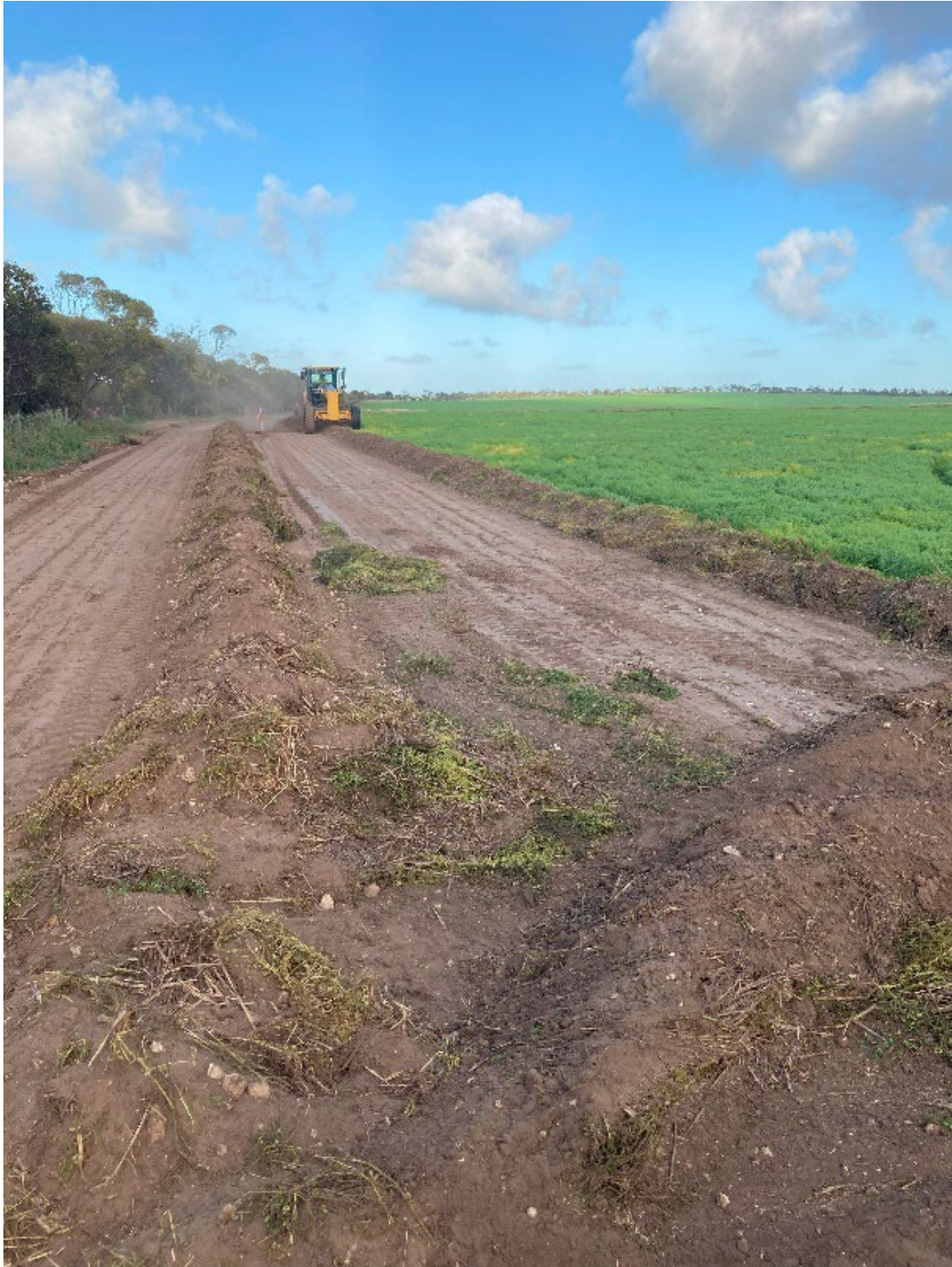
Figure 2: Site construction activity at the Ramsay Project Area
