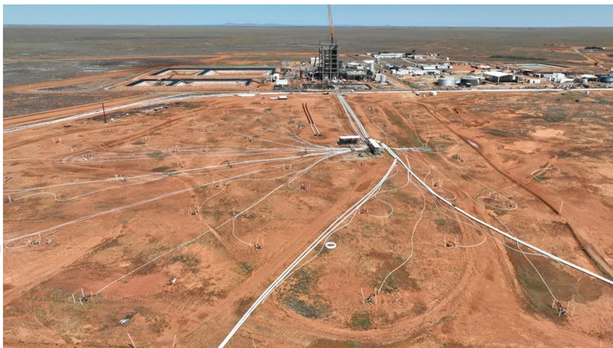
Image 1: Picture of the start-up wellfield prior to pre-conditioning and commissioning
