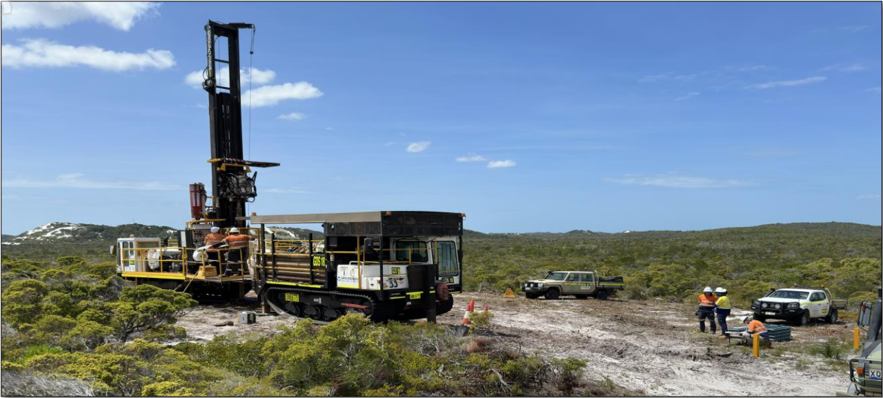
Figure 1: Sonic drilling rig completing groundwater bore drilling
