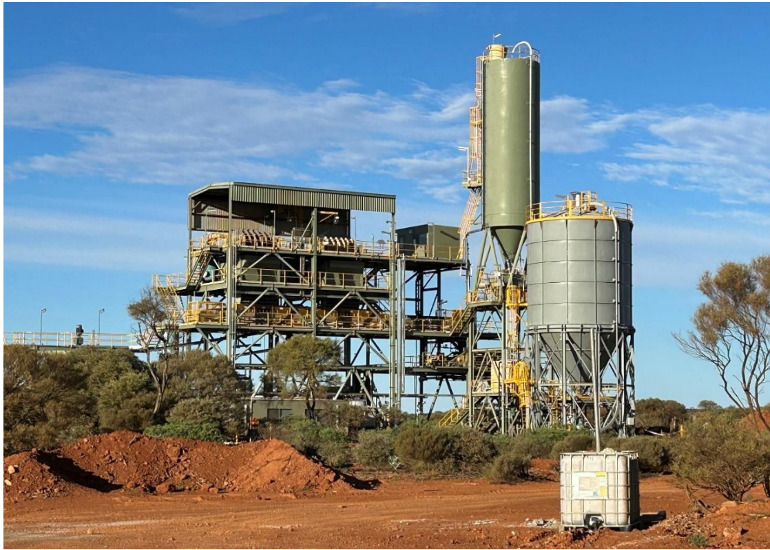
Figure 7 – Abra paste-fill plant.
