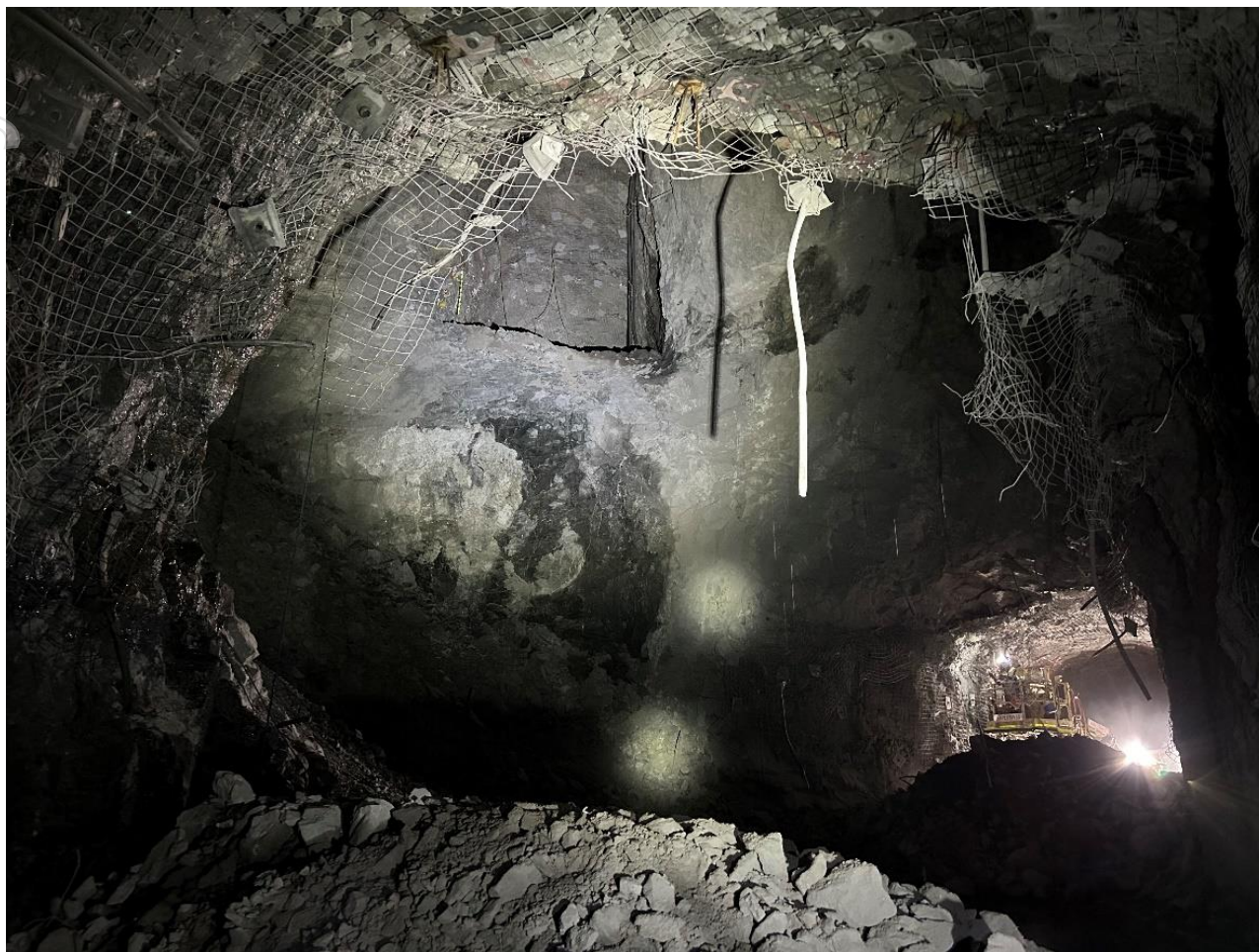
Figure 11 – Picture showing large underground stope at Abra on the 1280mRL level which will be paste filled in October after completion of mining (Photo 5 September 2023).
