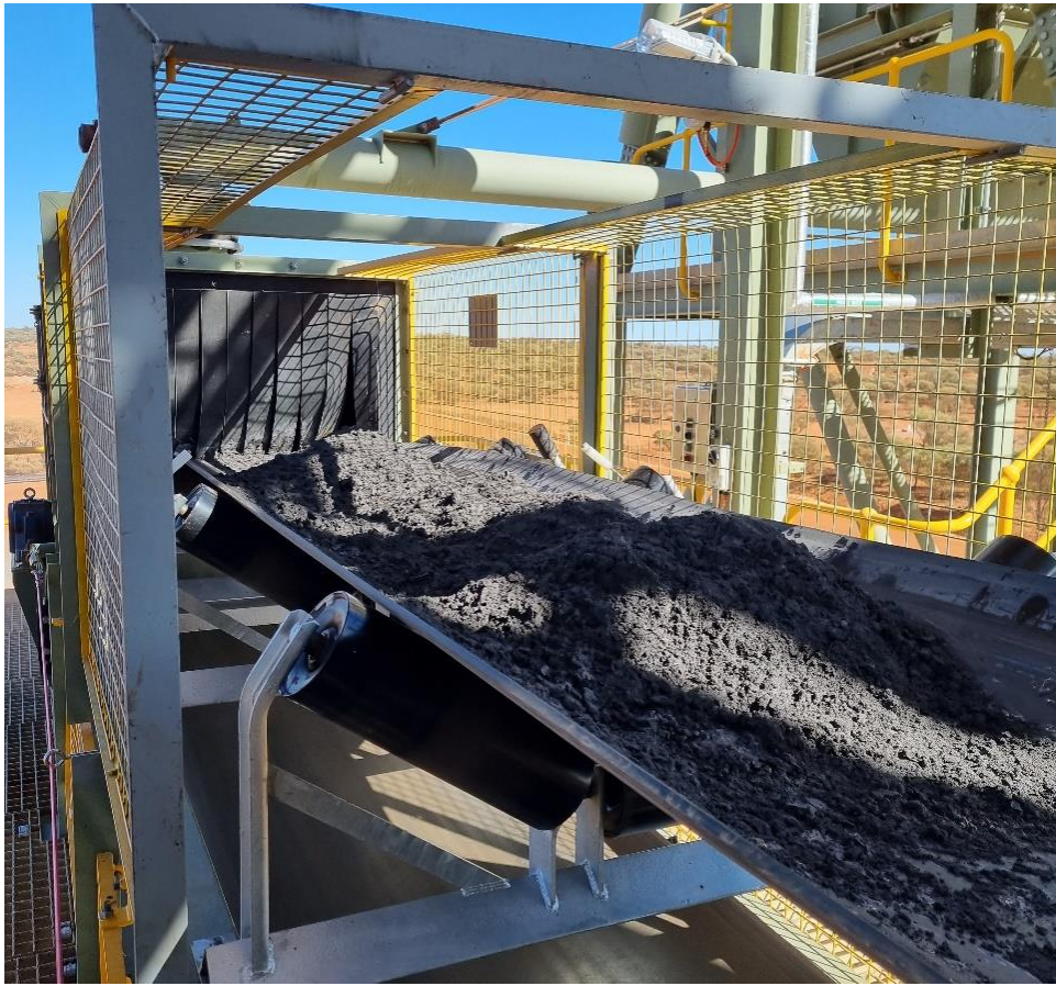
Figure 9 – Filtered tailings at Abra entering paste mixer prior to piping underground (Photo 5 September 2023).
