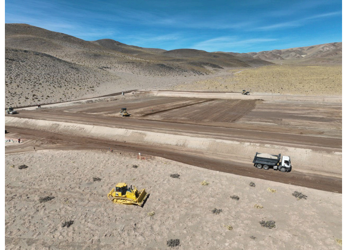
Figure 15: Construction of the First Evaporation Ponds at HMW
