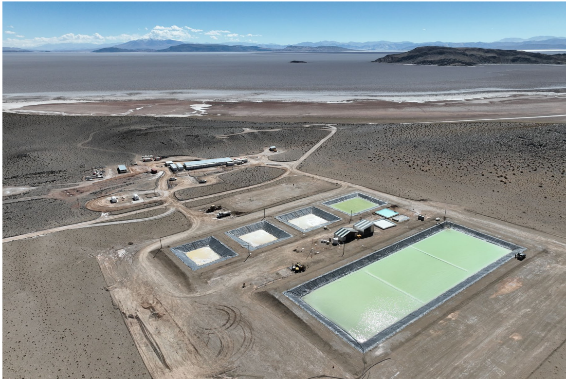
Figure 14: Pilot Plant at HMW
