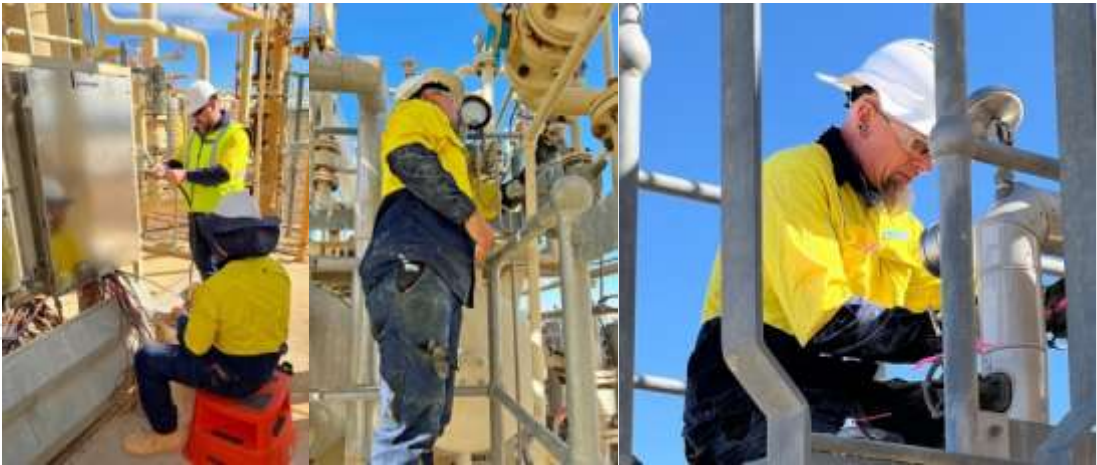
Refurbishment works underway at Eromanga
