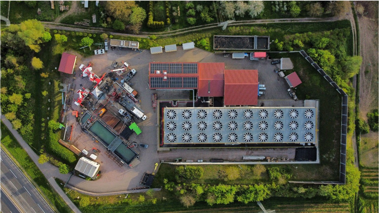
Figure 8 Aerial photograph of Vulcan's Natürlich Insheim Geothermal Plant.
