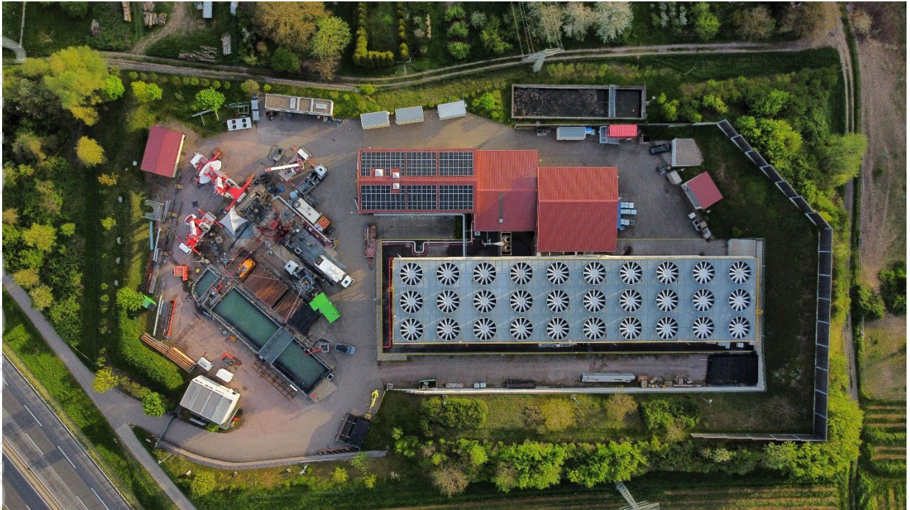
Figure 8 Aerial photograph of Vulcan's Natürlich Insheim Geothermal Plant.
