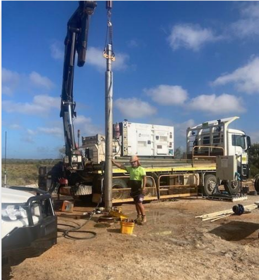
Figure 4: Bore testing equipment
