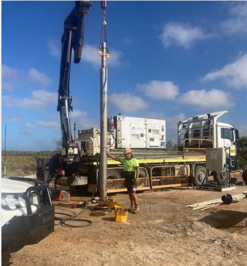
Figure 4: Bore testing equipment
