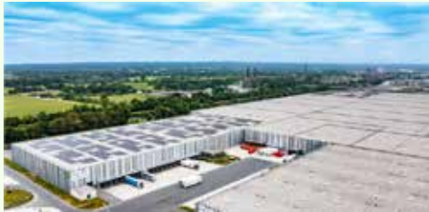
Goodman's largest solar installation globally Marl, Germany
