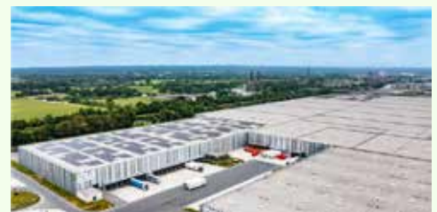
Goodman's largest solar installation globally Marl, Germany
