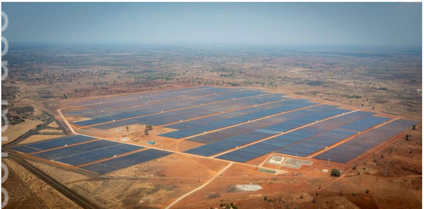
Figure 31: 60MW Salima Solar Power Plant in Malawi recently constructed and commissioned by JCM (source: JCM)
