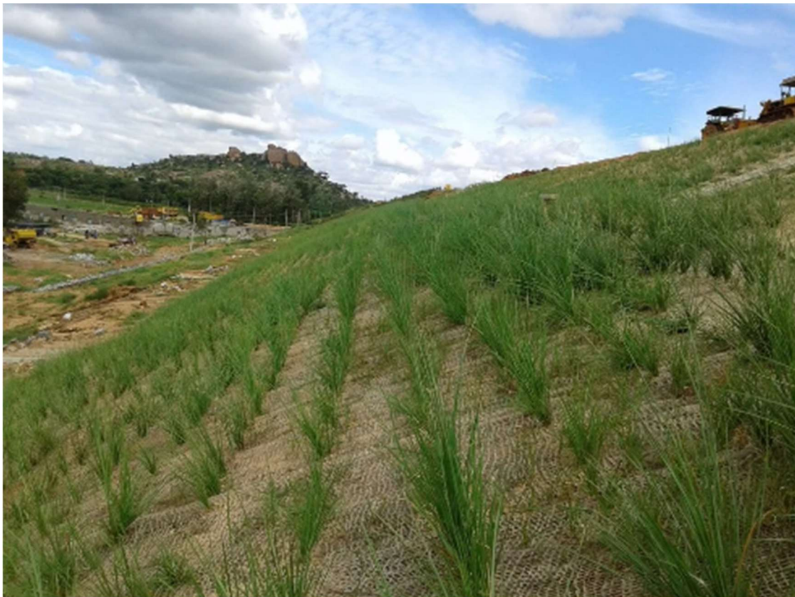
Figure 29. Example of a vetiver cover crop at a TSF rehabilitation site in southern Africa
