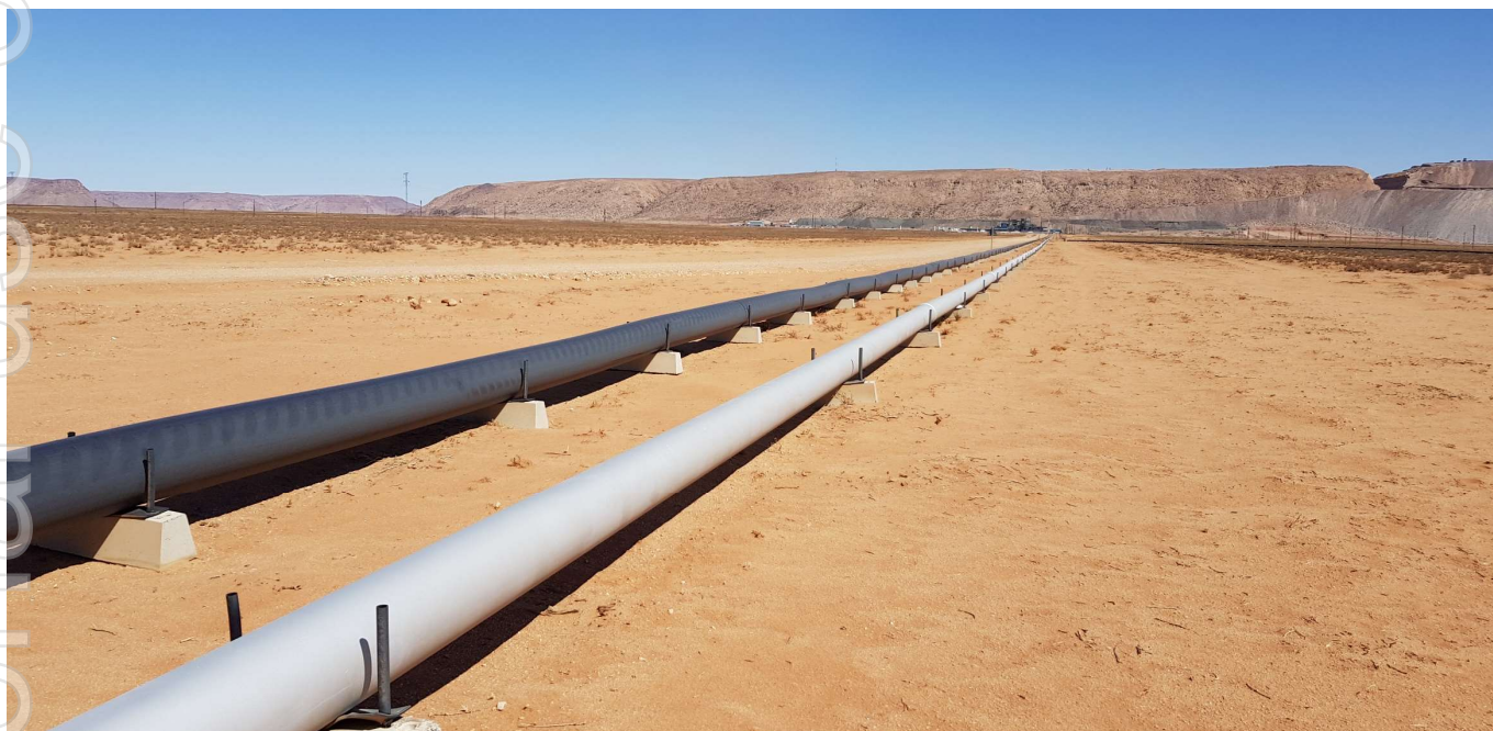
Figure 11: Example of overland pipes the concept planned for Kasiya (Source: Paterson & Cooke)
