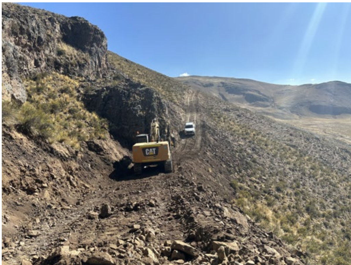
Figure 4: Access road construction underway at Picha Project in Peru
