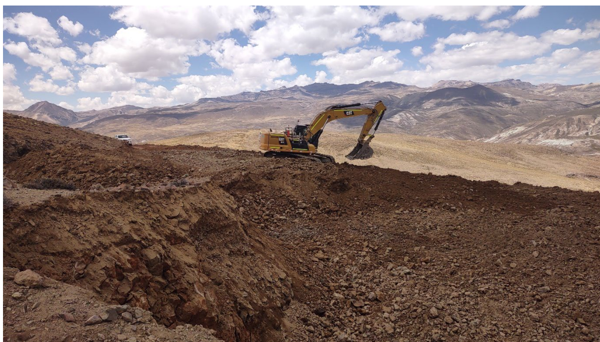
Figure 5: Drill pad construction underway at Picha Project in Peru
