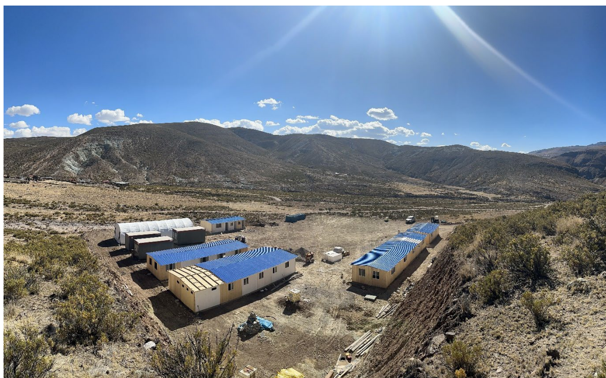
Figure 3: Exploration camp under construction at Picha
