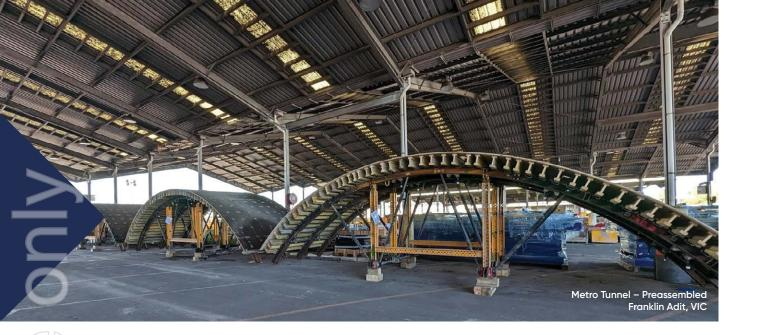
Our product versatility and solutions focus allows us to supply multiple added formwork packages and provide all engineering design, supply and preassembly.
