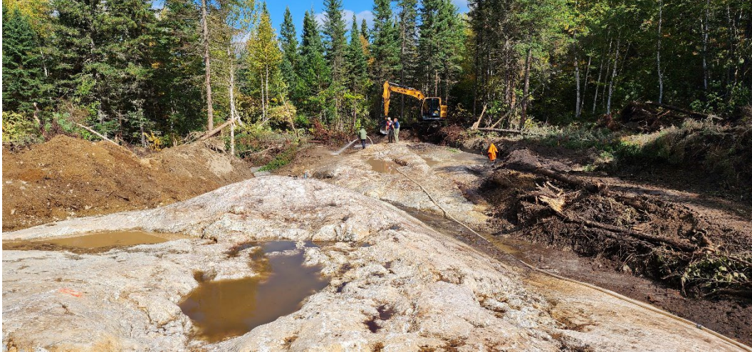
Figure 5 – Mechanical stripping underway at Nelson occurrence
