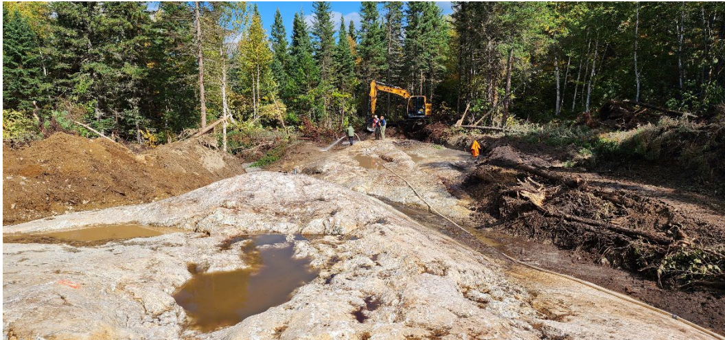
Figure 5 – Mechanical stripping underway at Nelson occurrence
