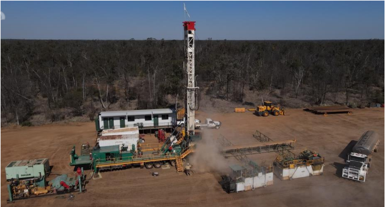
Water well drilling at Daydream-2 wellsite
