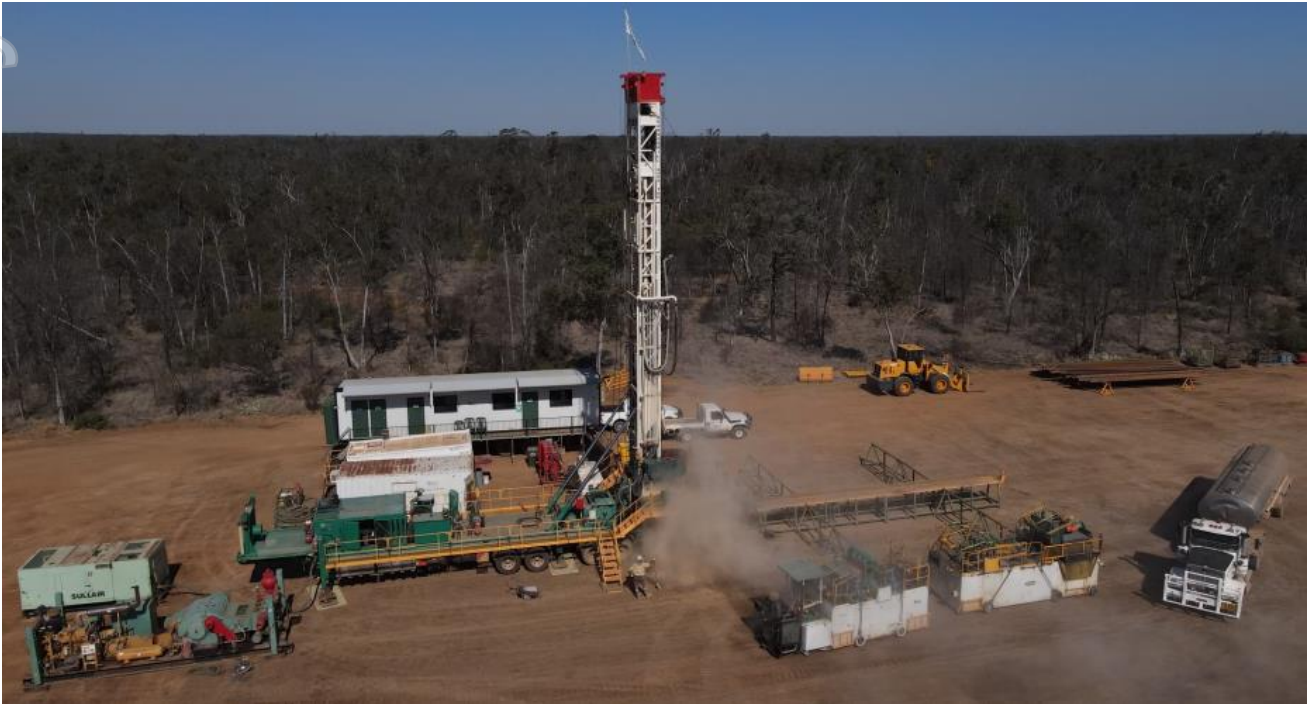
Water well drilling at Daydream-2 wellsite
