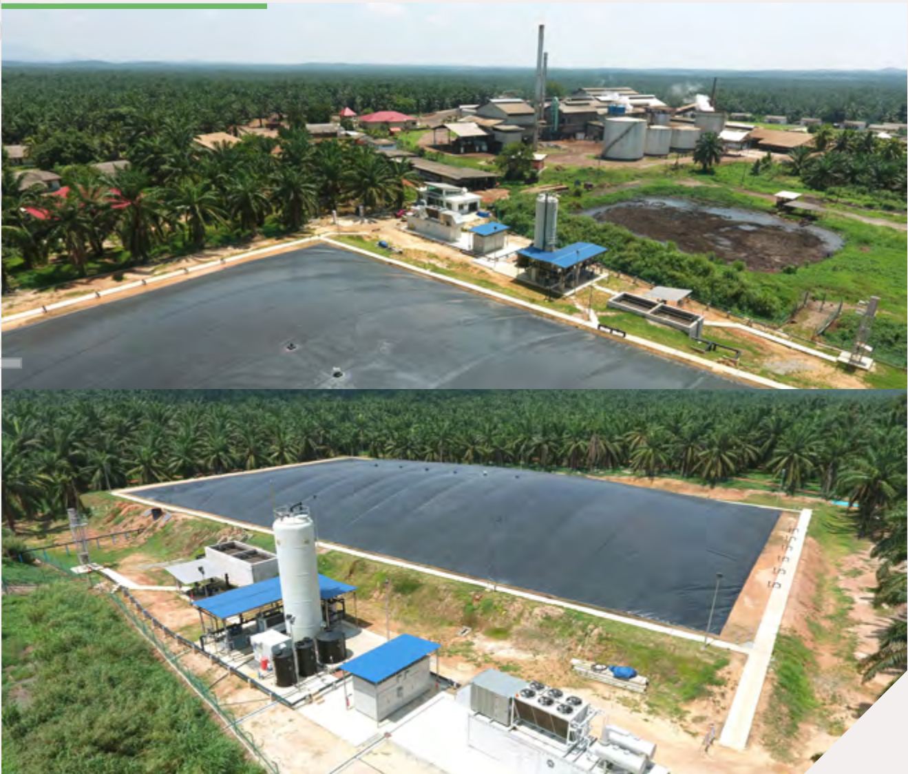
ABOVE Layout of Methane gas treatment plant and biogas engine station with covered lagoon in background.
