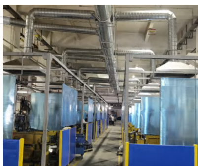
Newly installed weld fume and dust extraction system at an APG supplier
