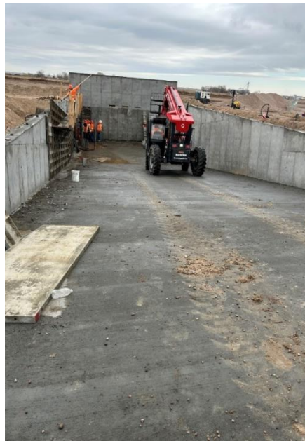
Figure 10. Longs Peak Dairy-fluid retention basin with walls.
