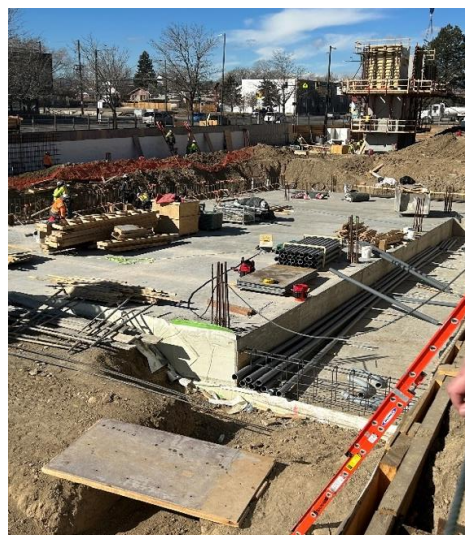
Figure 7. Installed foundations
