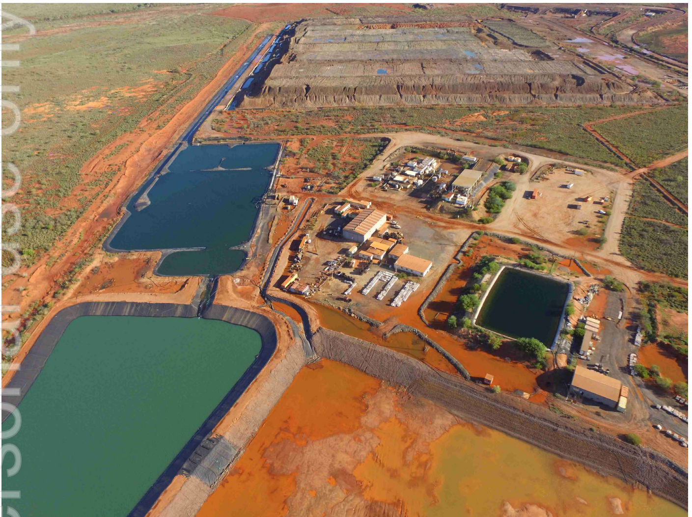
Figure 1: Whim Creek Heap Leach and Associated Infrastructure
