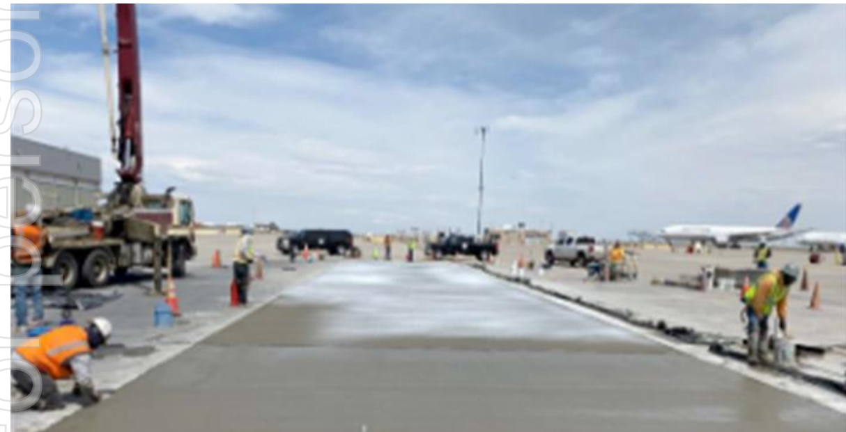
Denver Airport- concrete replacement -United Airlines
