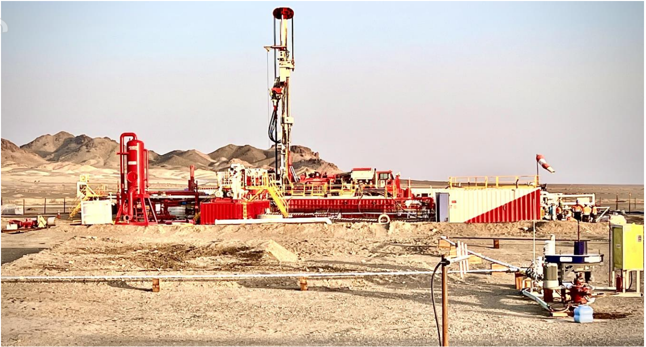
Drilling Rig at Nomgon-10
