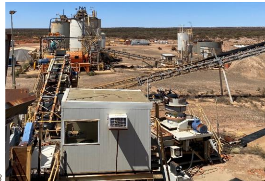
Laverton Processing Plant. May 2023
