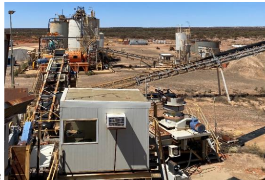
Laverton Processing Plant. May 2023
