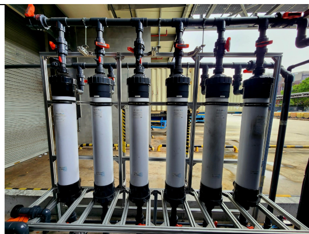
Image 2) De.mem Ultrafiltration membranes as key component of overall BOO plant
