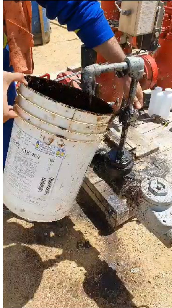
First look at oil from Unit-1B
