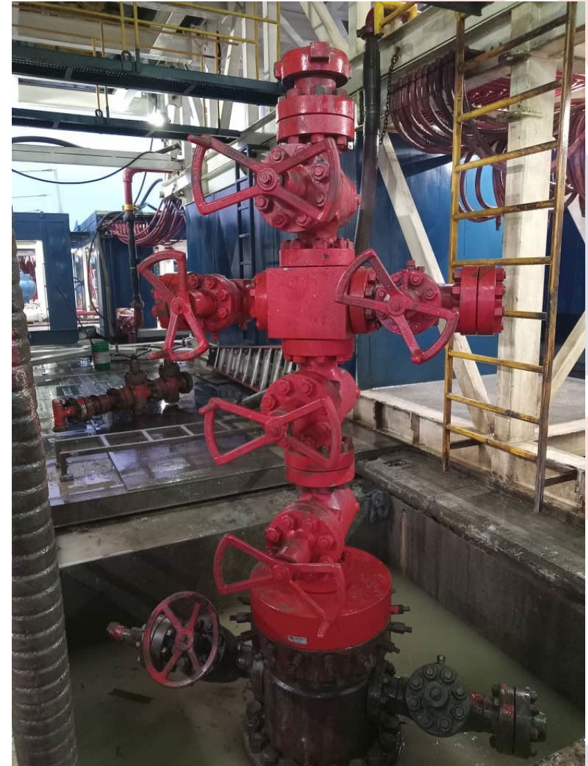
Alameda-2 Completions Ran Successfully
