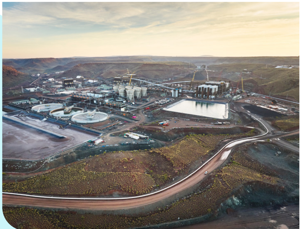
Iron Bridge Project
