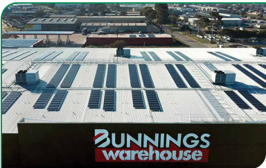
Bunnings' hundredth on-site solar PV system
