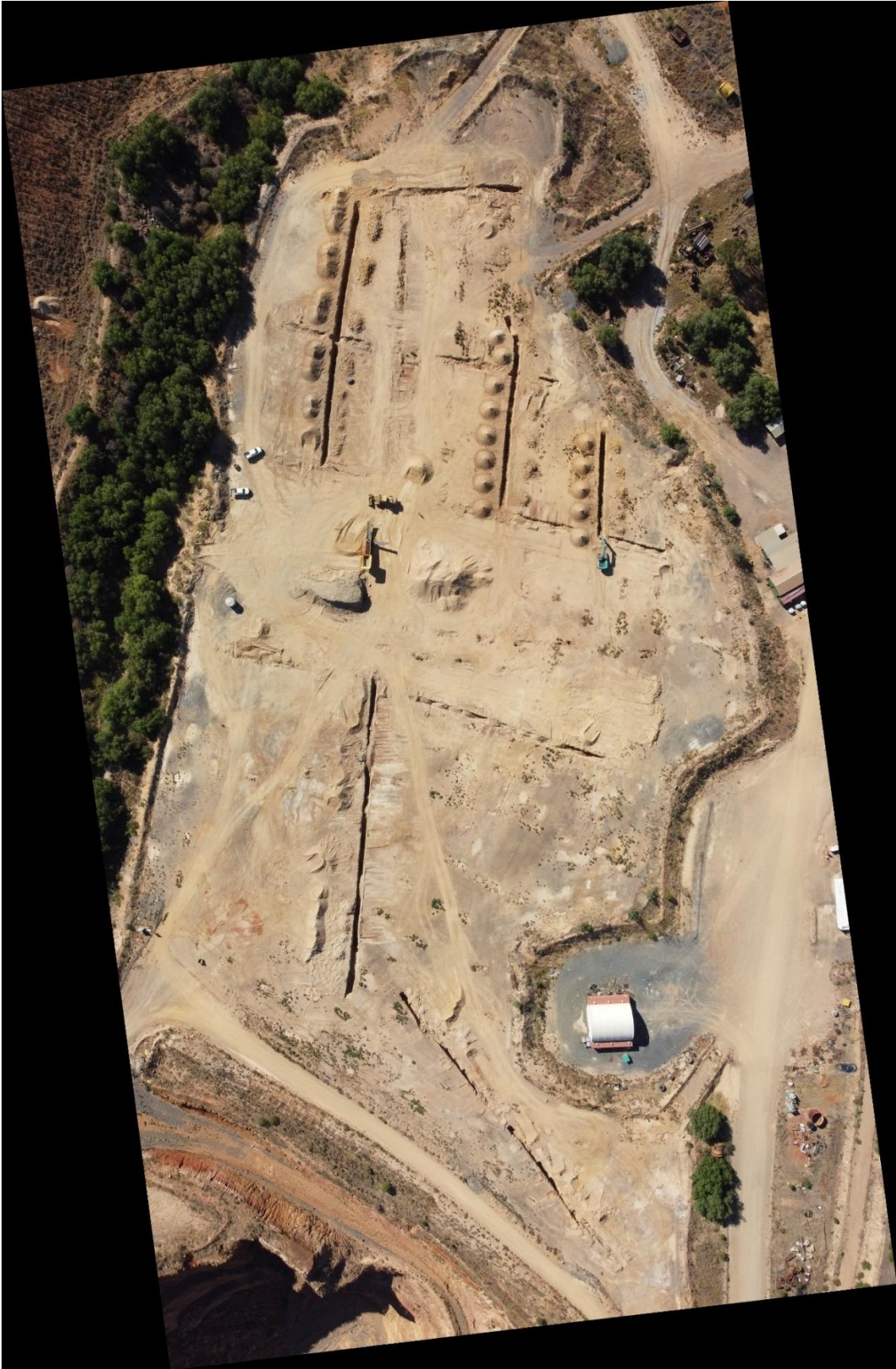
Figure 1: Drone view of Trench evaluation of the Mt Boppy ROM rock dump and tailings
