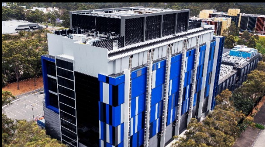
Macquarie Park Data Centre Campus Intellicentre 2, Intellicentre 3 East Intellicentre 3 Super West
