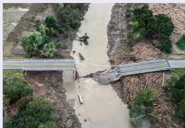
Damage to the regional fibre route on the bridge crossing the Hikuwai River, north of Gisborne, required 800 metres of fibre to be overlaid.
