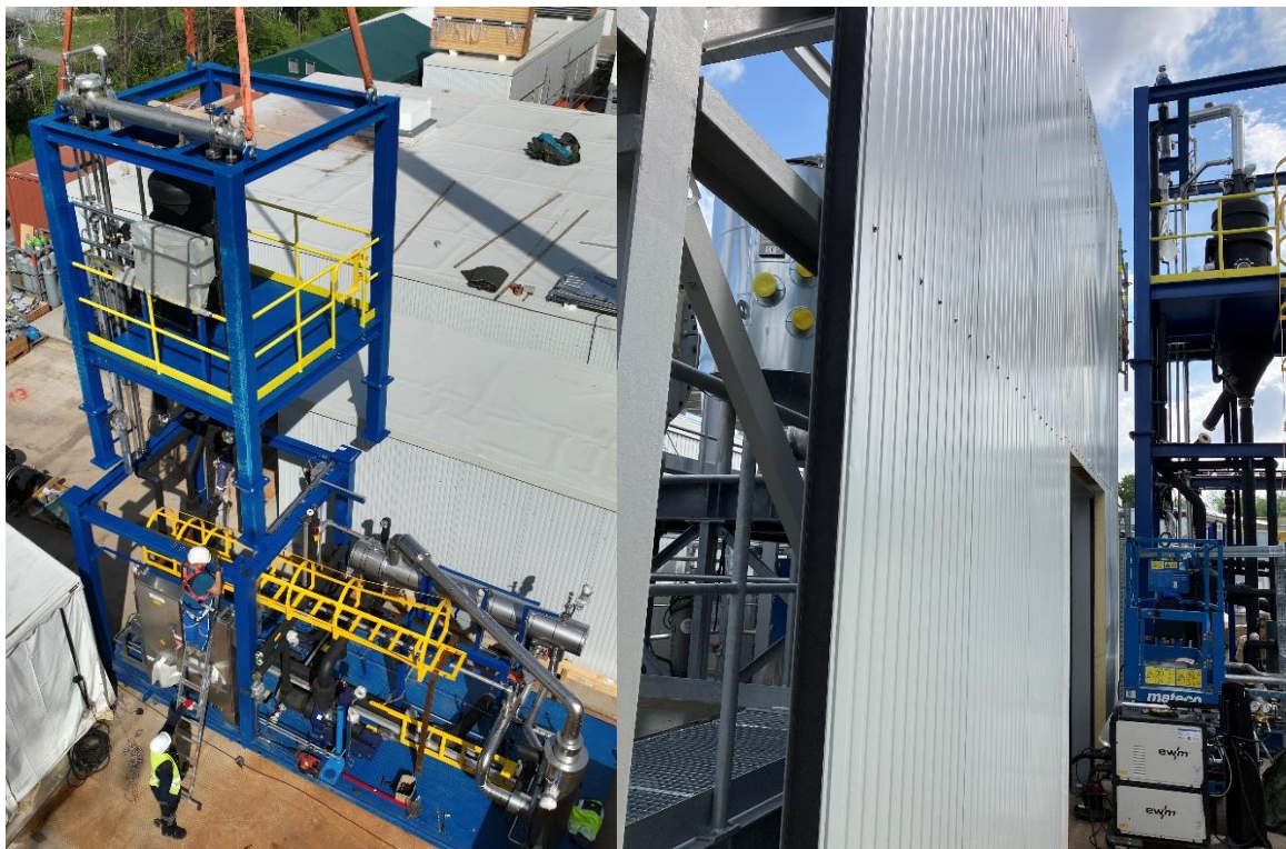
Figure 2 and 3. Crystalliser installation
