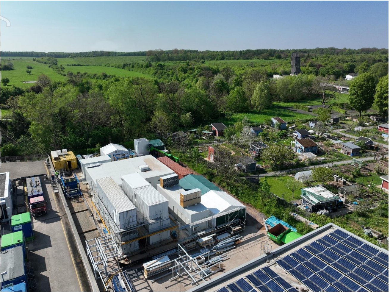
Figure 1. Vulcan's Lithium Extraction Optimisation Plant at Landau
