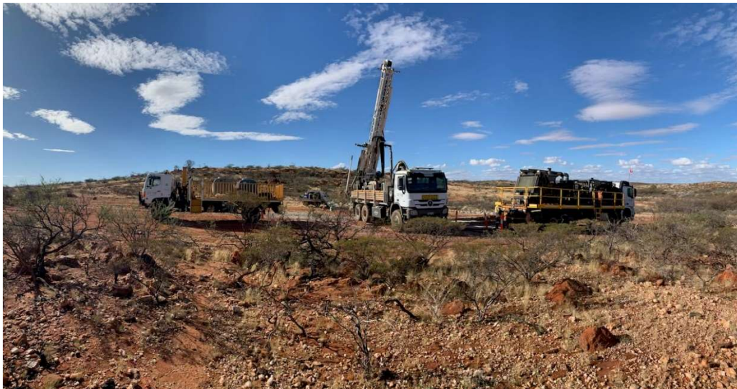
Figure 1: One of the drill rigs on site
