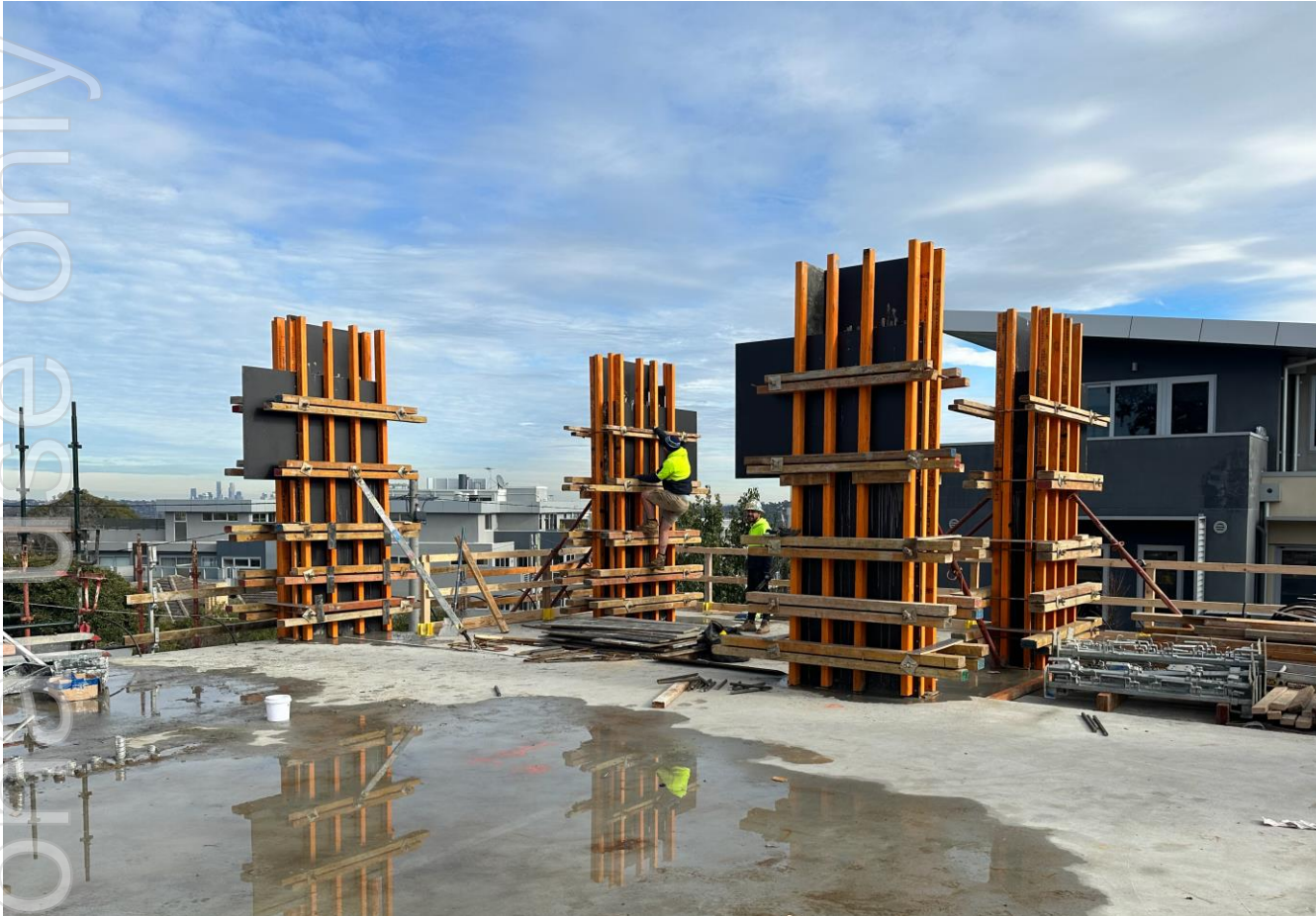
Genius Childcare - under construction, Templestowe Lower, Vic
