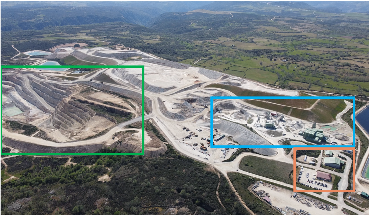
Fig.2 - Barruecopardo Site: In Green shown the mining operation, in Blue shown the crushing & screening circuits and main processing plant; in Orange shown the laboratory and administration building
