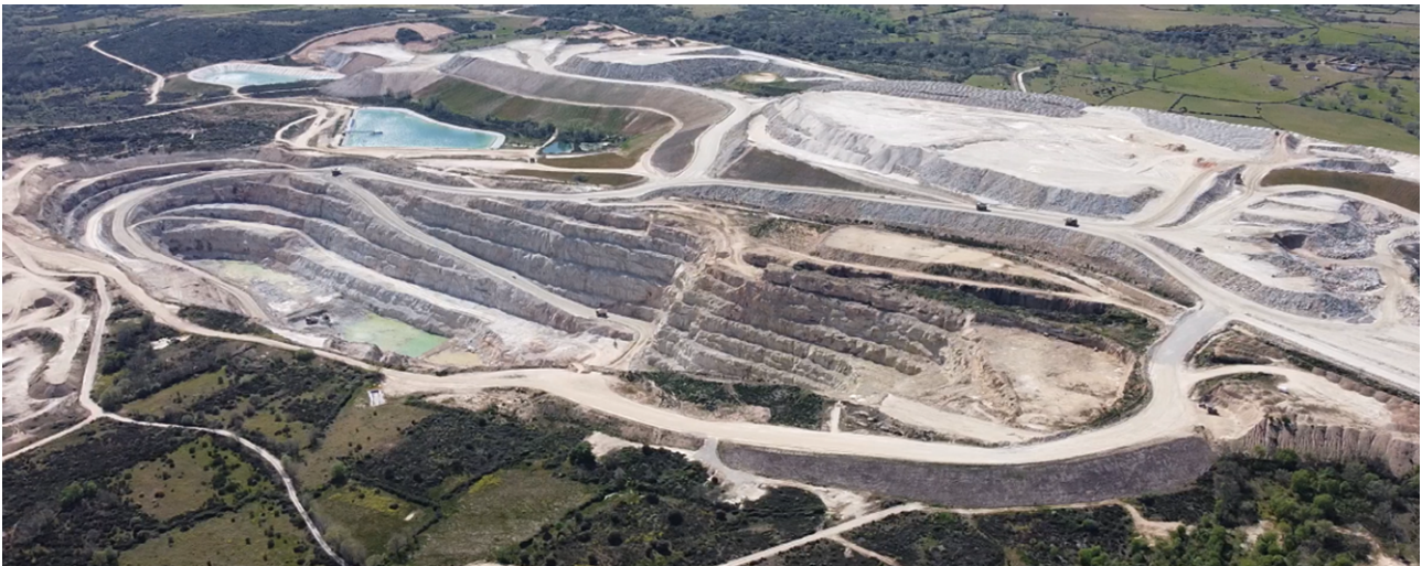
Fig.4 - Aerial view of the Barruecopardo open pit (as of July 2023)
