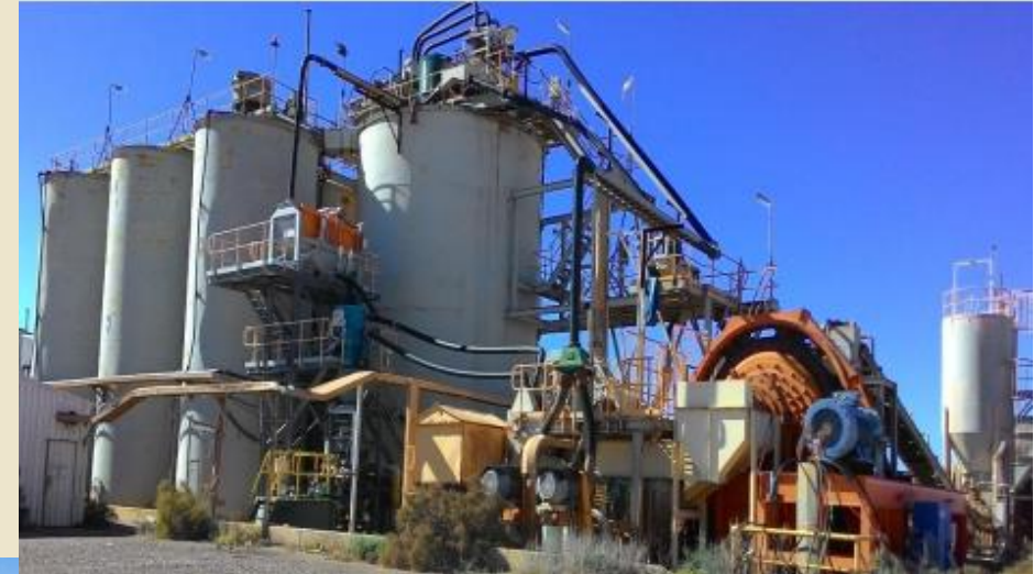
Processing Plant & Infrastructure in Laverton
