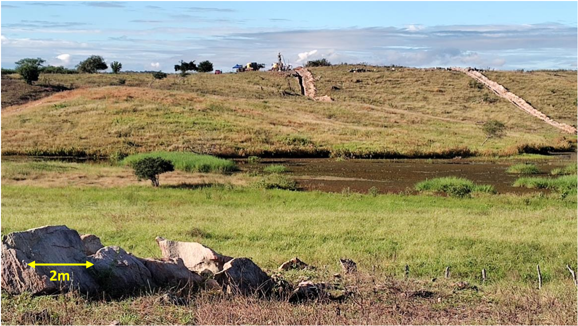
Photo 4 – Drill Rig at top of hill at end of trench at Rolados
