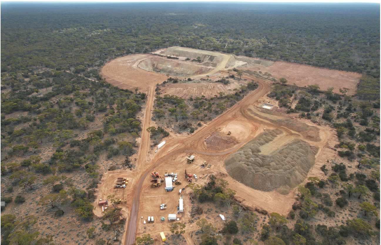
Jeffrey's Find Mine site.
