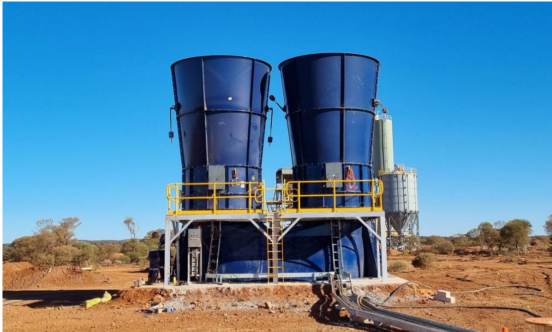
Figure 2 – Successful installation of the second primary ventilation fan at Abra during July on the mine’s primary 6m diameter exhaust rise (Photo 25 July 2023).
