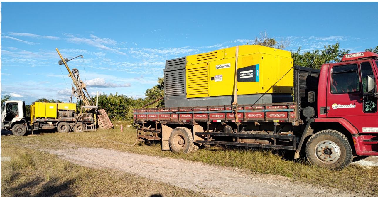
Photo 2: Drill rig advancing inclined Hole RC-011
