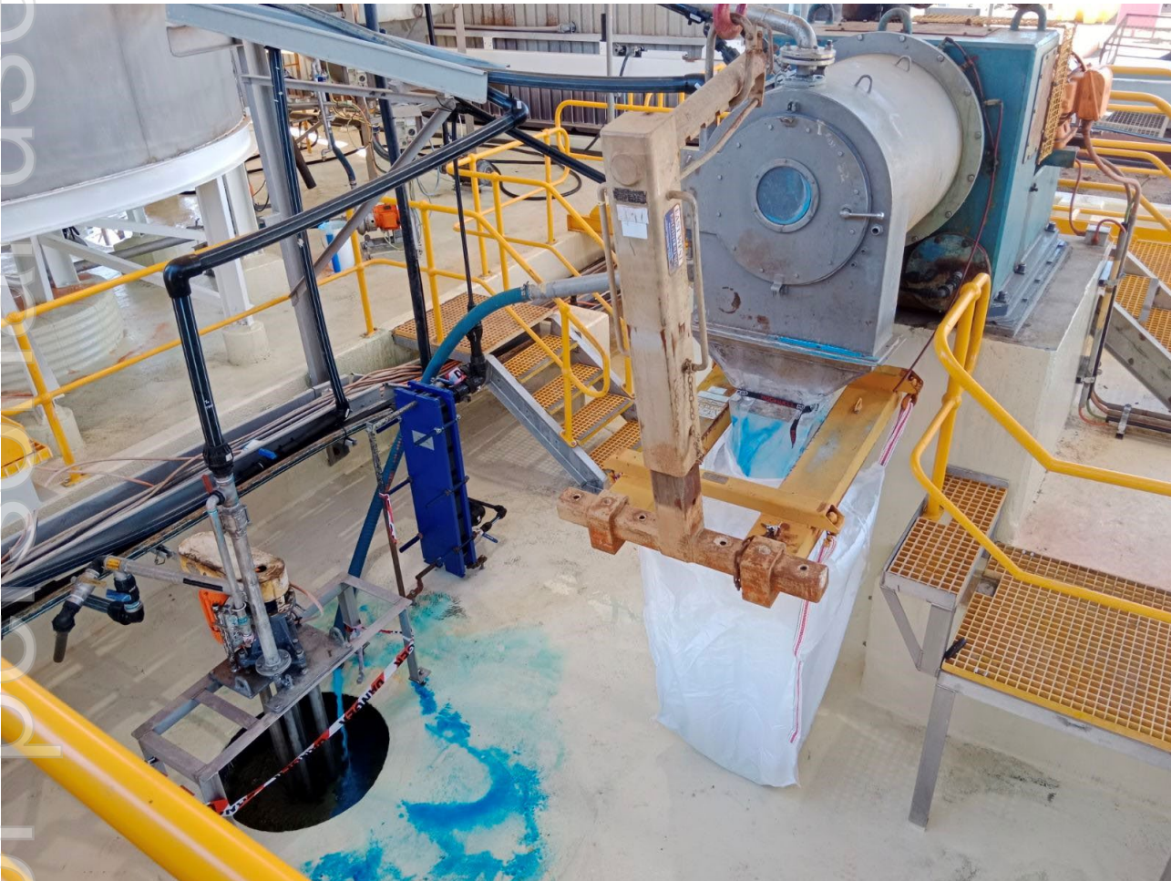
Figure 1: Copper sulphate crystal loaded into a Bulka bag from the plant centrifuge at the Cloncurry Project Copper Sulphate Plant
