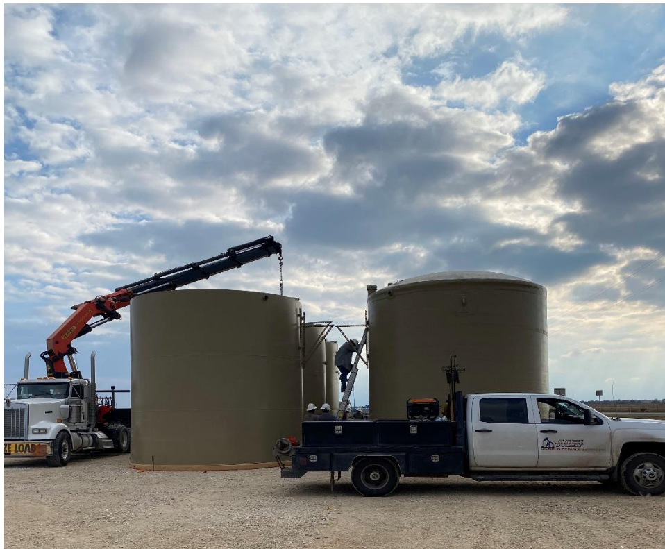
Figure 1: Varn Facilities Installation
