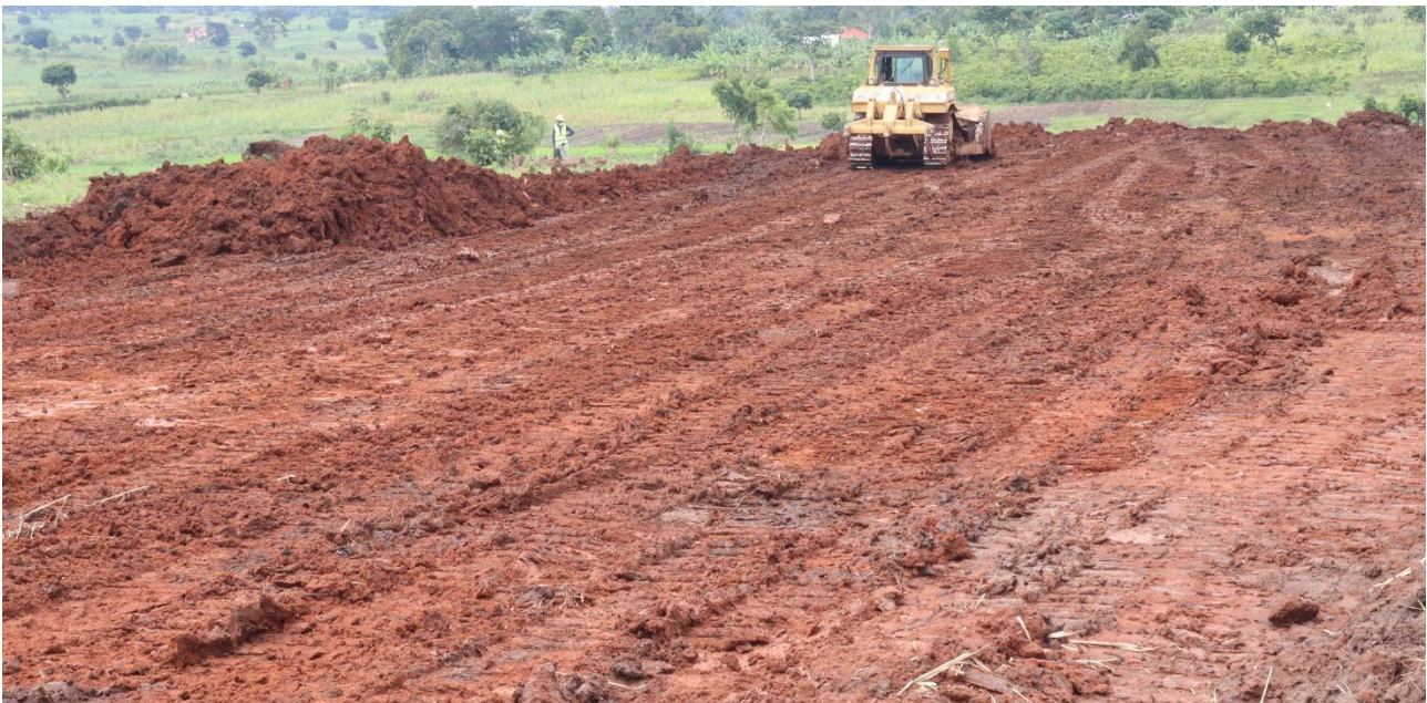
Figure 2: Demonstration plant earthworks progressing at the site of where the Makuutu Demonstration Plant Technical Facility will be located.
