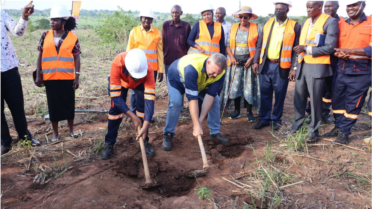
Figure 1: Makuutu Demonstration Plant ground-breaking performed by RRM Country Manager, Patience Singo (left), and Ben Vietnieks (ADT Africa, Right) along with Bugweri District officials at the Makuutu Demonstration Plant site in the Makandwa Village, Makuutu Sub-County.
