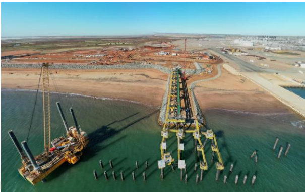
Jetty piling completed
