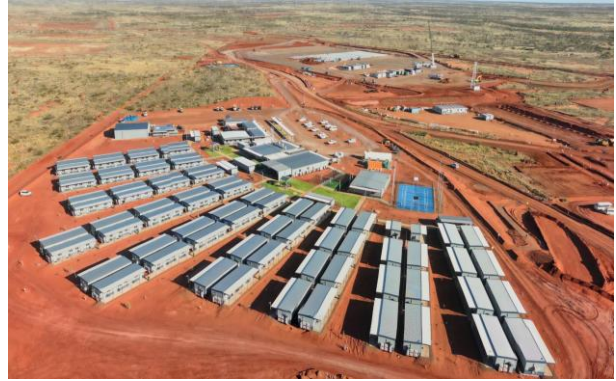
Onslow 300 room construction camp completed
