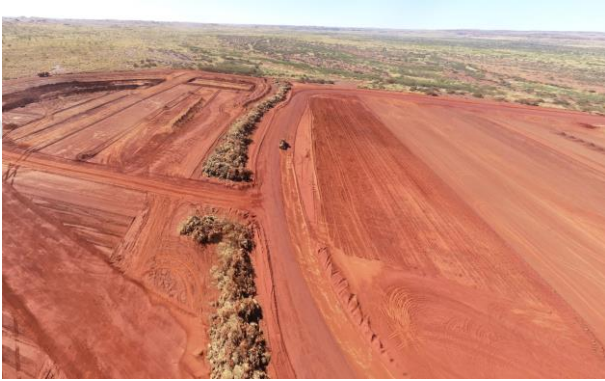
Clearing for resort style accommodation
