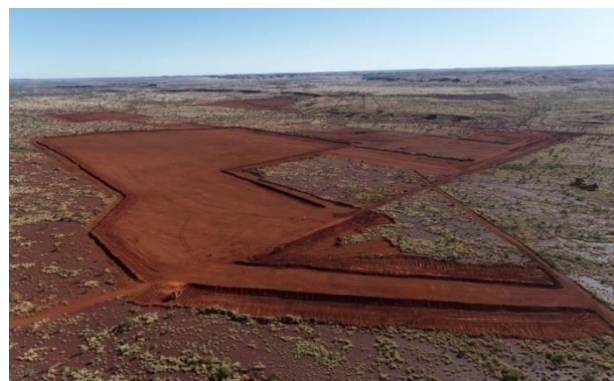
Crushing area cleared
