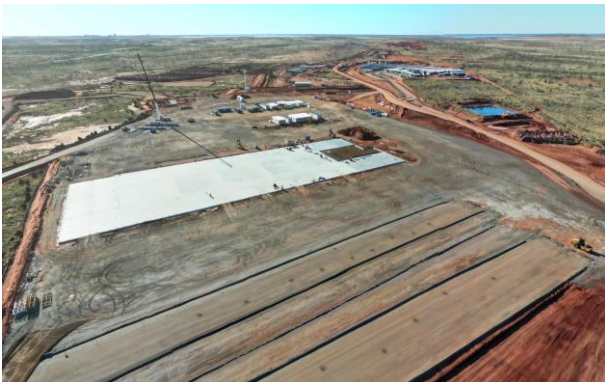
Construction of Truck Maintenance Facility
