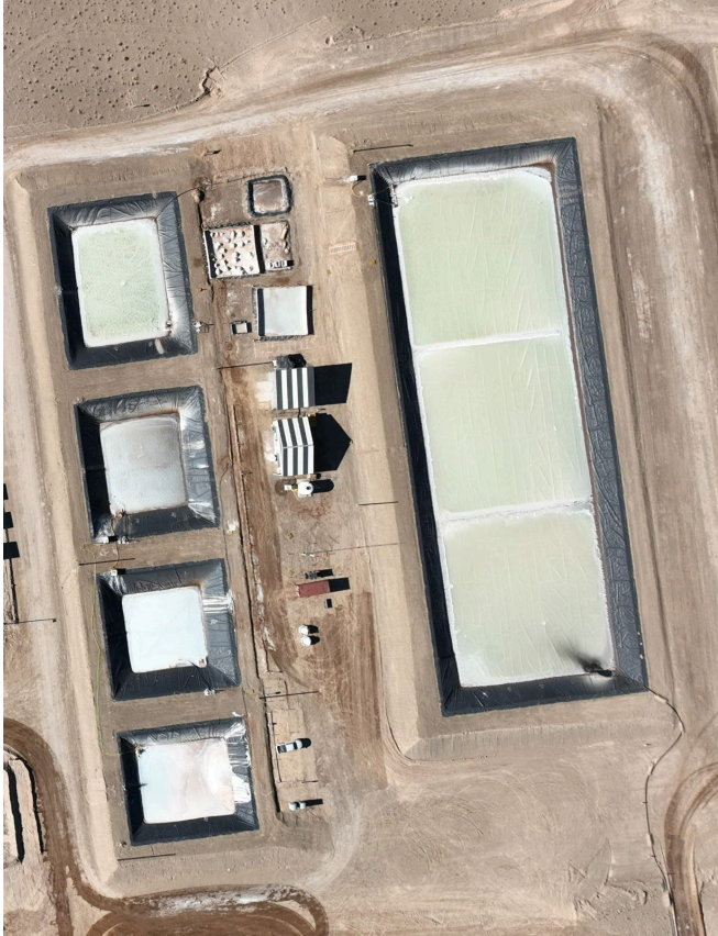
Figure 4: Aerial view of existing pilot plant
