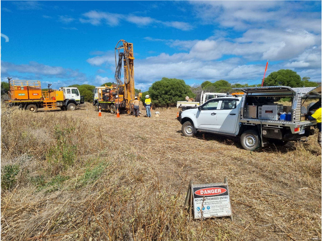
Figure 5: Bostech drilling rig on site
