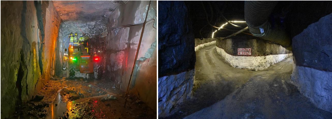
Figures 1 and 2: Underground Development on Kundu
