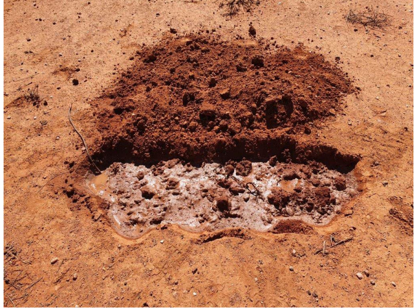
Digging and watering pit for electrode and prepared electrode in the ground
