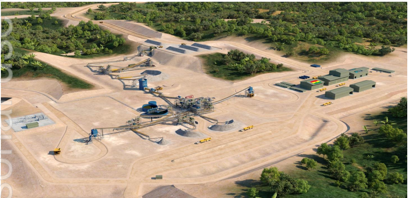
FIGURE 8 PROCESSING PLANT AND INFRASTRUCTURE VIEWED FROM THE WEST.
