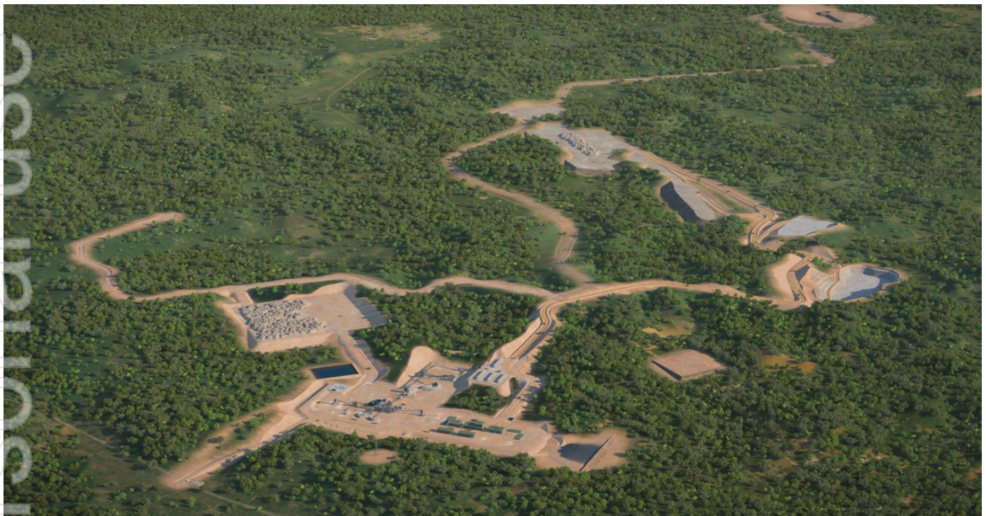
FIGURE 1 SITE OVERVIEW LOOKING NORTHEAST, YEAR 1 OPERATION
