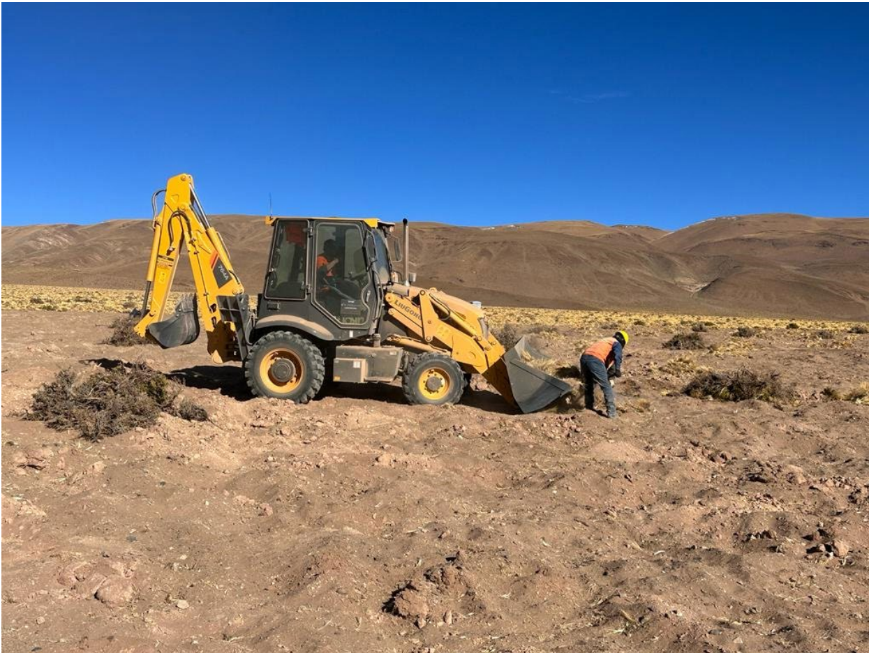
Commencement of top-soil removal at HMW
